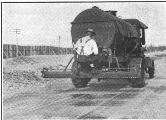
Huge oil-sprinkler mounted on motor truck for Sioux City track
